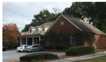
Existing medical office
