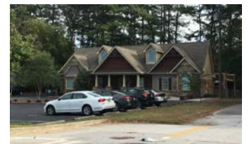
Existing medical office
