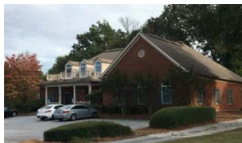
Existing medical office
