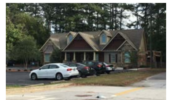
Existing medical office
